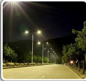
STREET LIGHTS & 24 HOURS ELECTRICITY
